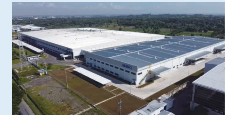
New factory building at PT. ISEKI INDONESIA (right)
