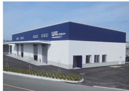
Large maintenance and service facility (Mashiki town, Kumamoto prefecture)
