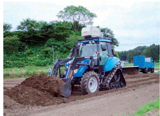
Decontamination work with TJV85 tractor
