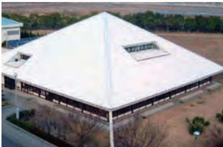
Full view of welfare facility
