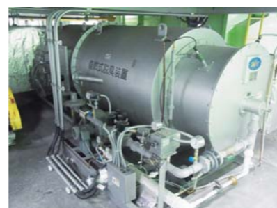
LPG burner for the drying furnace
