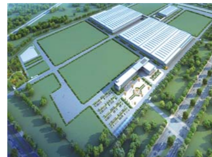
New plant in Xiangyang, Hubei province
