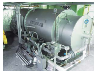
LPG burner for the drying furnace
